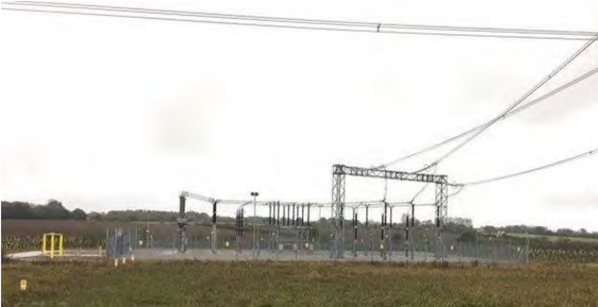
Figure 3.7 - Example Cable Sealing End Compound with gantry
