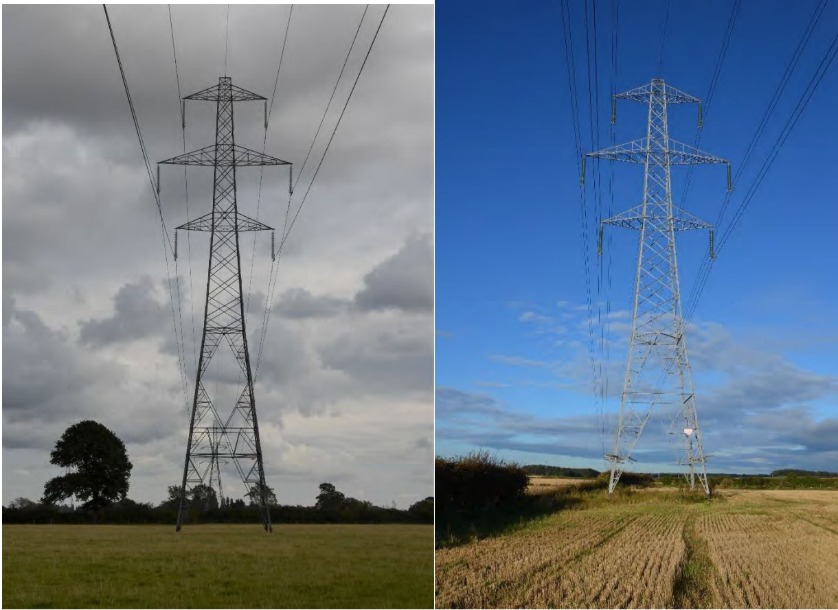
Figure 3.14 – Example of single conductors (left image) and twin conductors (right image)
