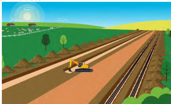
Step 7 The topsoil is reinstated on top of the trenches and the site access removed
