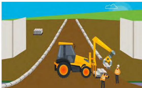
Step 3 Kerb lines would be installed along the edge of the bellmouth
